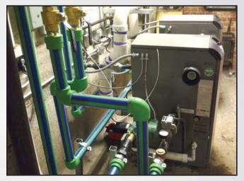
controlling the steam valve on the hot water converter. "We simply moved the wire into the lead boiler and programmed it to control the modulation rate of the cascade. I didn't even have to adjust the PID controller, and the system maintains reset setpoint to within plus or minus 2 degrees...smooth as silk," Smet continued.
